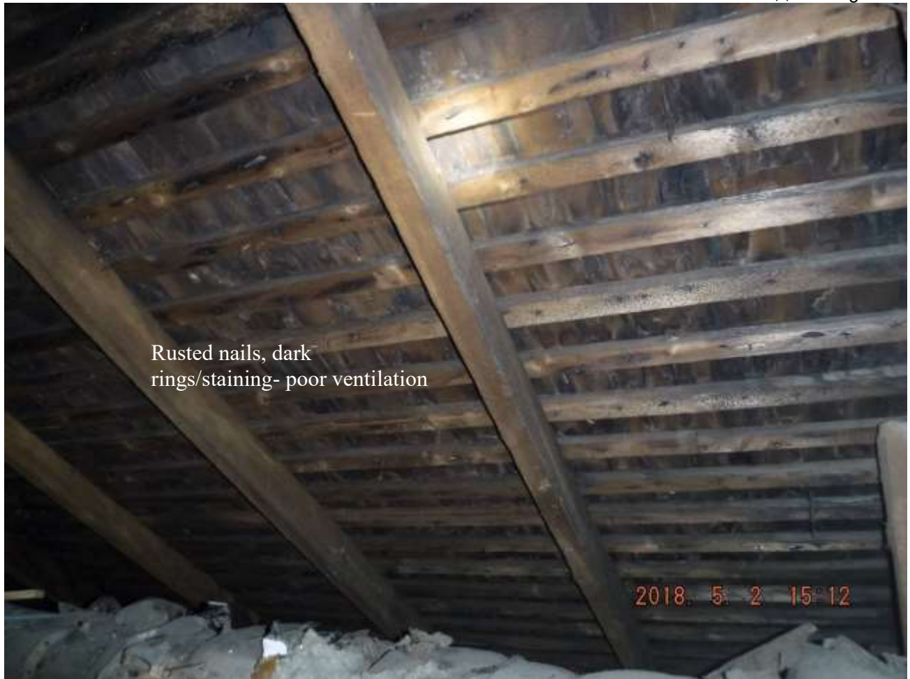
Figure 4 Cedar shingles under asphalt shingles, rusted nails, no collar ties, poor ventilation, etc. Roof is past its life and has structural concerns. Recommend a structural engineer (PE), roofer and or building contractor further evaluate roof & structure and advise on structure repairs, roof replacement, ventilation & insulation and gutters.
