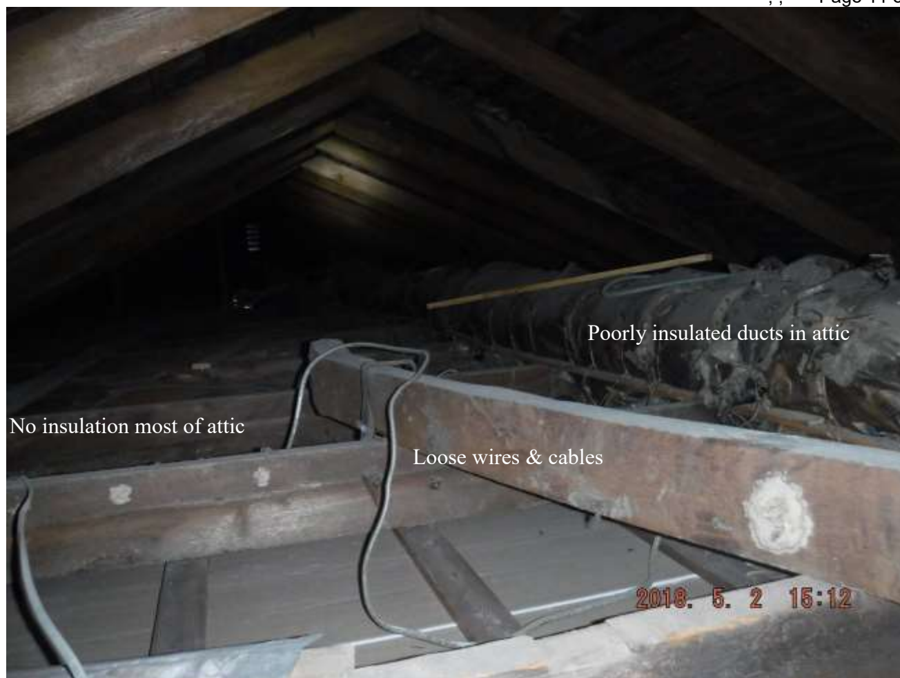
Figure 2 Main front section of attic; no insulation, poorly wrapped insulation on ducts and loose wires. Roof structure was substandard and had deficiencies and past expected life.
