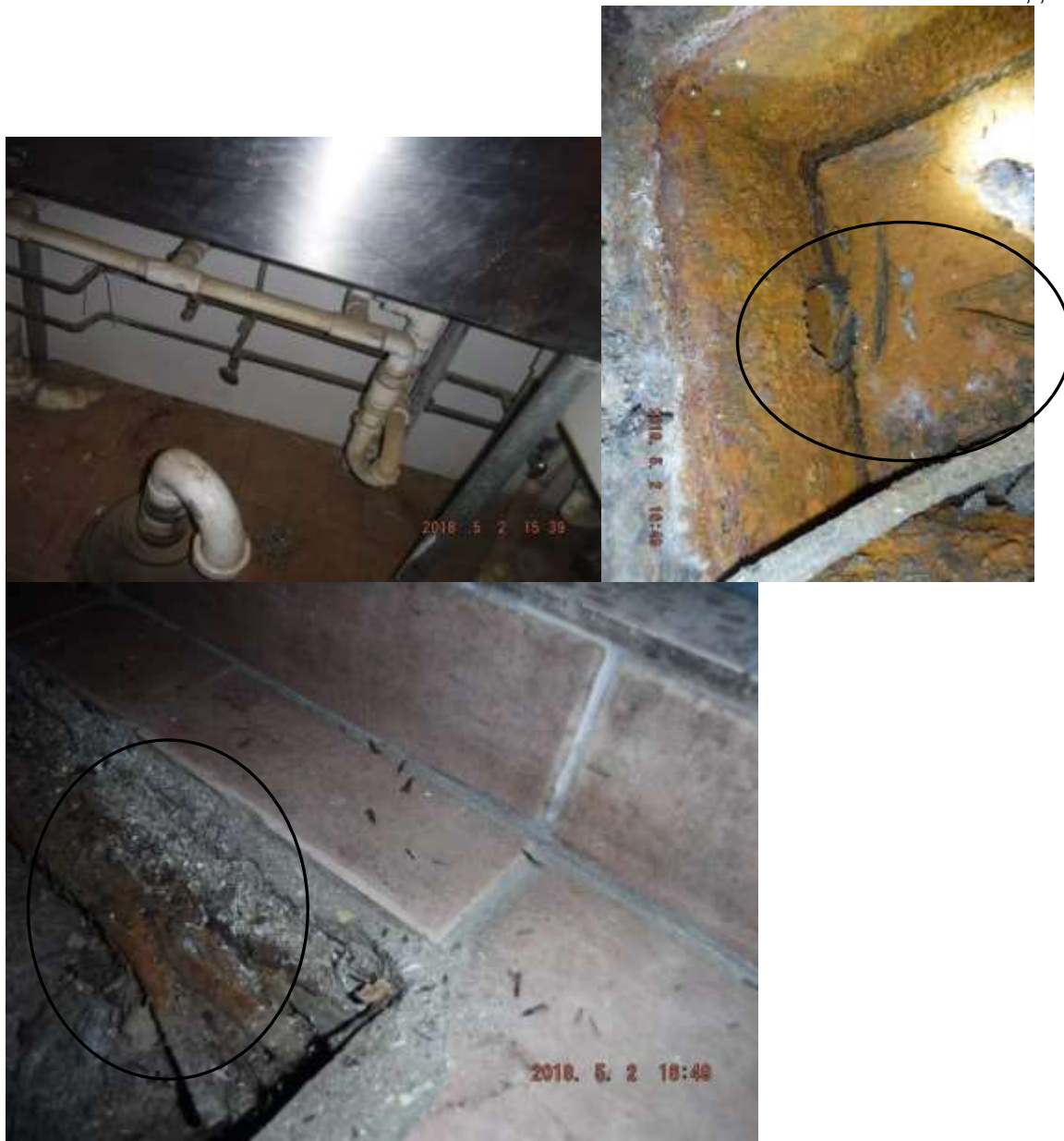
Figure 10 Rusty floor trap and termite swarmer wings & body parts.
