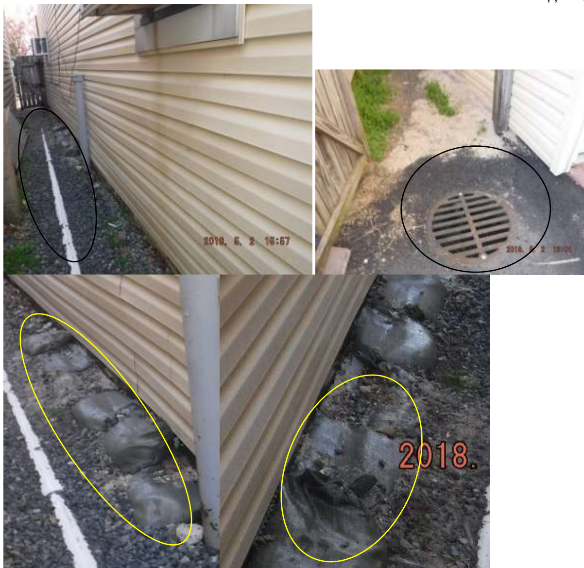
Figure 1 Follow up with Clinton boro to see if they maintain and service the drains in alley; not tested or accessible. There were several sand bags around the slab foundation and neighboring stores; indicative of flood measures.
